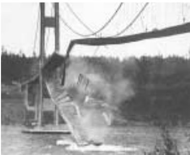
Tacoma Narrows Bridge Failure
